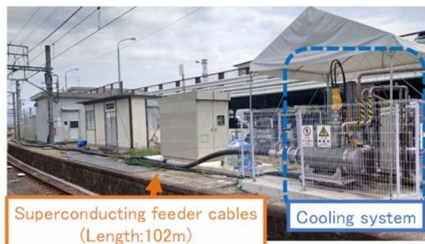
Fig.1 Superconducting feeder systems installed to commercial lines
