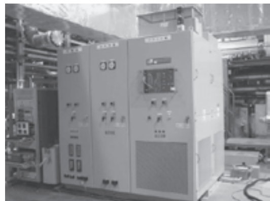
Fig.2 FCL panel board in which the cryostat, the compressor, and the circuit breakers are mainly installed
