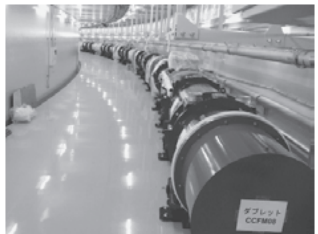
Fig.2 Superconducting combined function magnets installed in the J-PARC neutrino beam line.
