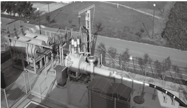
Fig.1 Photograph of the KEPCO HTS cable system.
